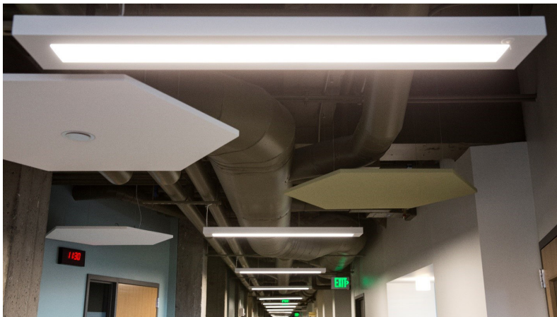
The Enlighted lighting controls system was the ideal choice for building system integration and lighting flexibility.
